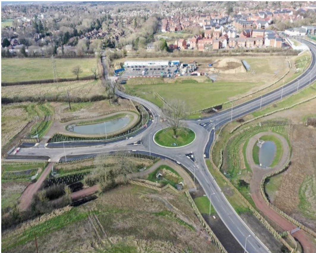
Figure 2-10 - New sections of Road and Roundabout along with new water drainage systems at ground level.
